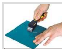
step 1: make grid cutting on surface
